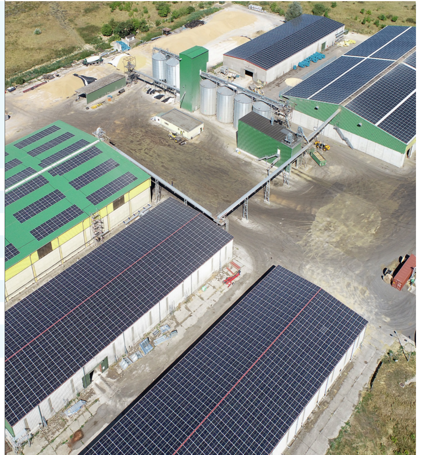
As part of the installation, 5,400 square meters of asbestos-containing roofs were renovated
